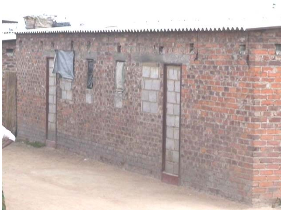
Photo 7: there are 18 government-funded, "Operation Garikai" houses in Hopley farm, Harare, where 3,800 displaced live: windows and doors have been bricked up because there are no door or window frames, and also no sewerage, water or electricity, five years after being built. [July 2010]
